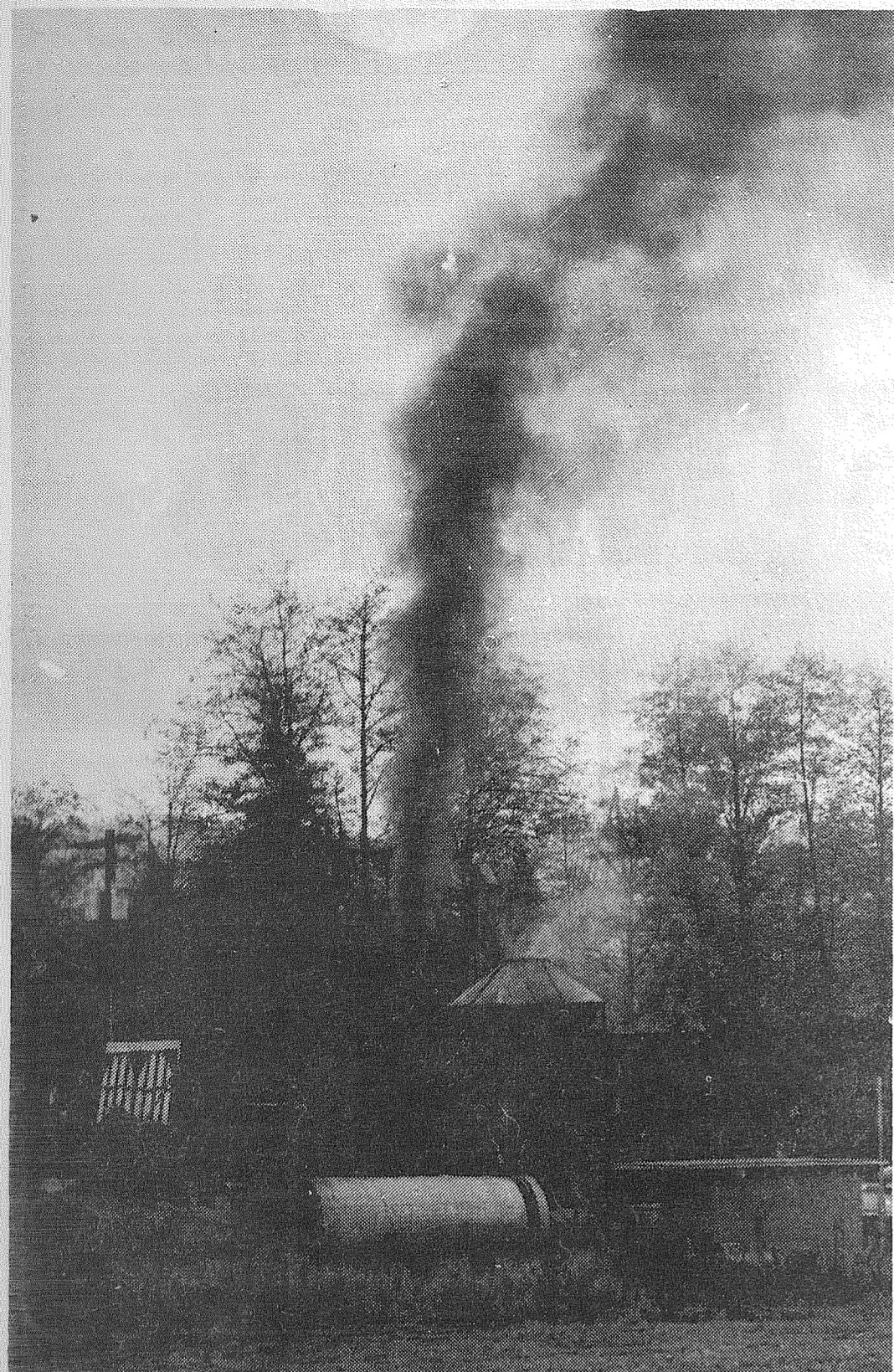
OIL BURNING BOILERS such as that on this small plant near Puyallup operate quite inefficiently and contribute to the smoke and smog which often settles in the Valley and elsewhere in Puget Sound. Smoke volume of one such boiler is not great, but each one helps contribute to the problem.
