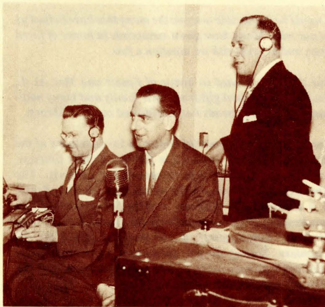
Radio staff at work in tower radio room
