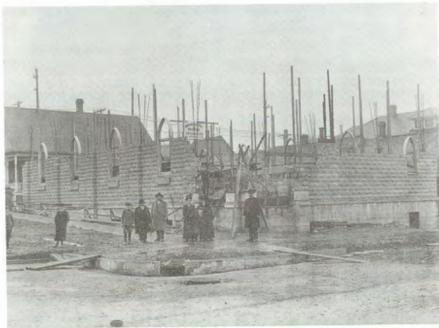
St. John's English Lutheran Church under construction 1908
