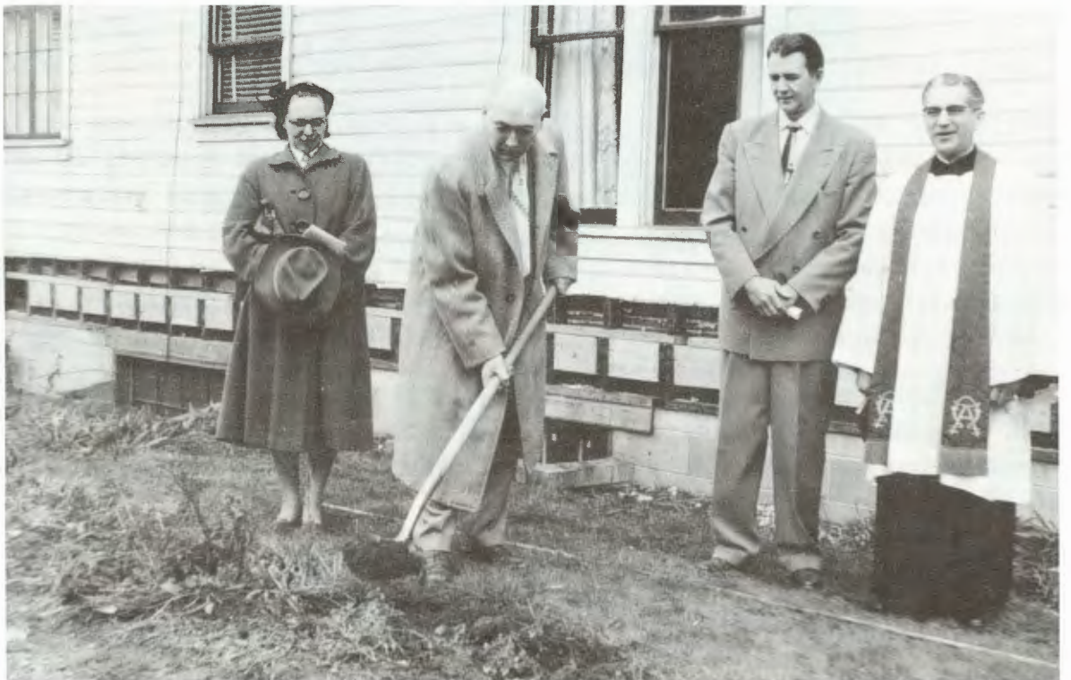
Ground breaking for Educational Building
