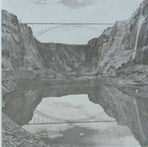
Glen Canyon damsite and bridge. The graceful steel arch bridge is 700 feet above the river.
