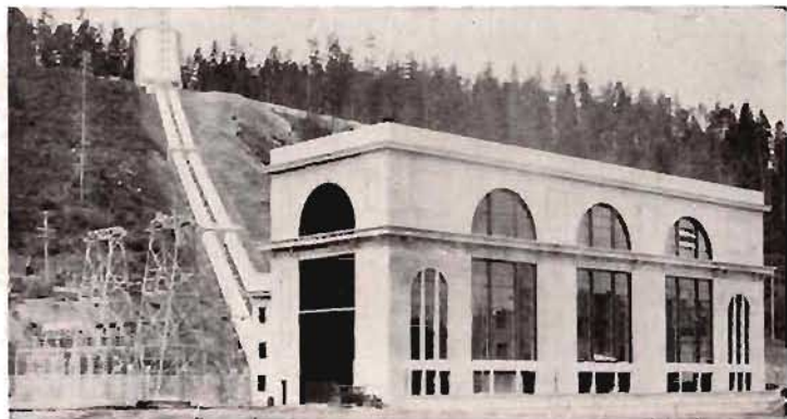
CUSHMAN POWER HOUSE No. 2 POTLATCH, WASHINGTON
