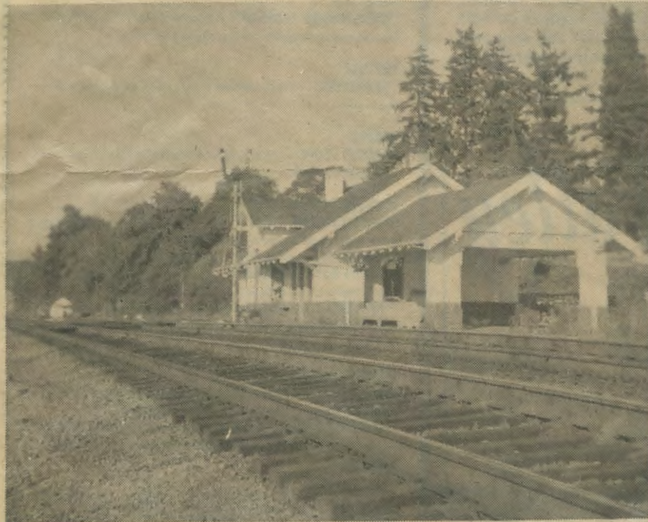
THIS OLD STATION, built when the Northern Pacific came to Steilacoom in 1914, may soon be torn down. The town had high hopes for becoming a rail terminus in the 1870's but lost to Tacoma. When the tracks finally came through they forced a drastic rearranging of the buildings and destroyed the once popular beach.
