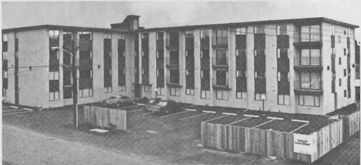
Most recent apartment project completed by Sandvig Construction 44-Unit - 1207 N.W. 92nd St., Seattle, WA 98117
