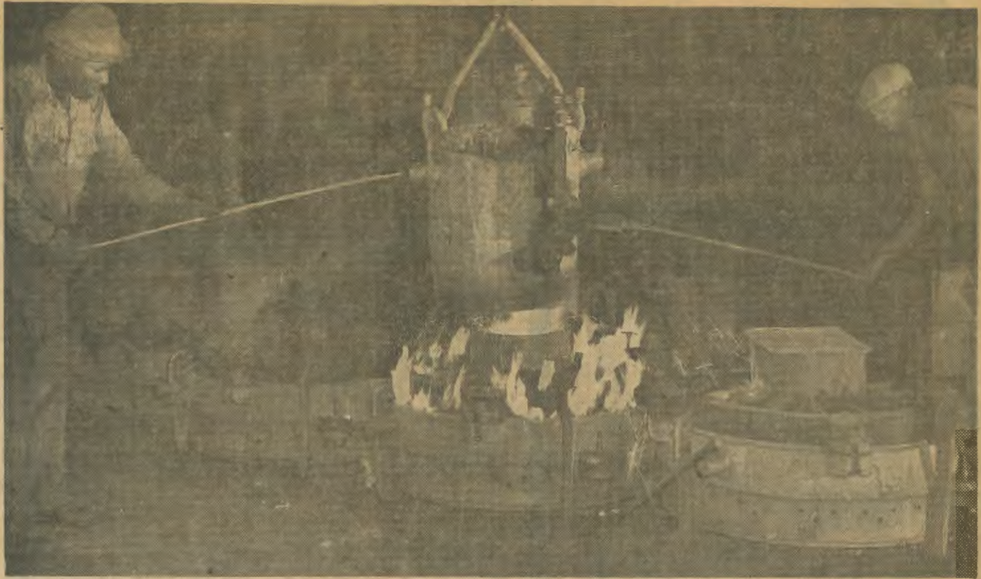
CHILLED CASTING —Casting of Griffin cast iron wheels took three days from the initial pour until they were ready for service. Two foundrymen for the Griffin Wheel Co., which closed last December, are pictured as they poured the molten iron into the wheel mold. The sudden chilling of the metal as it came into
