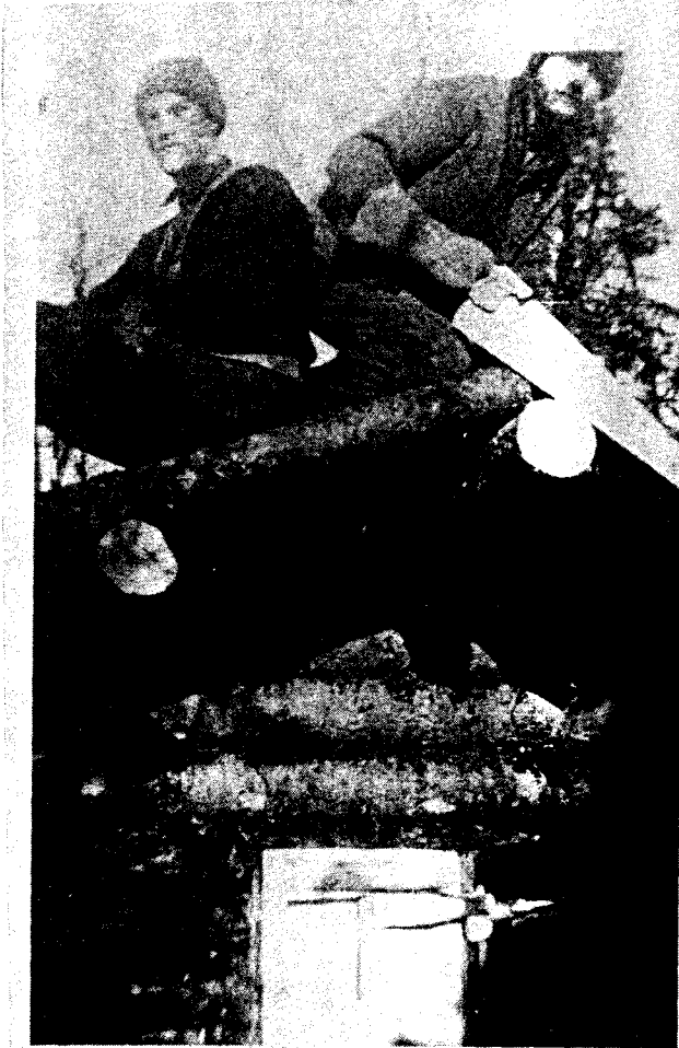
(Left) Carl, on the left, and Oscar, on right, just finishing work on the Beaver Point Cabin. =====
