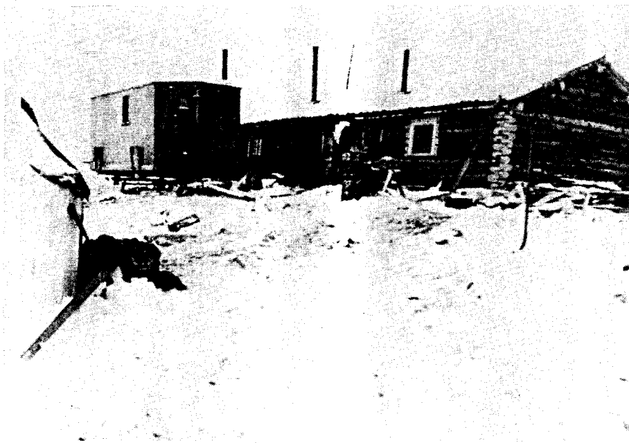
(Left) "Our house out at the mine. Wanagan standing on sled out front. Taken day before we started to the highway," Carl wrote referring to trip back to highway to haul more supplies to Blue Lead Extension.
