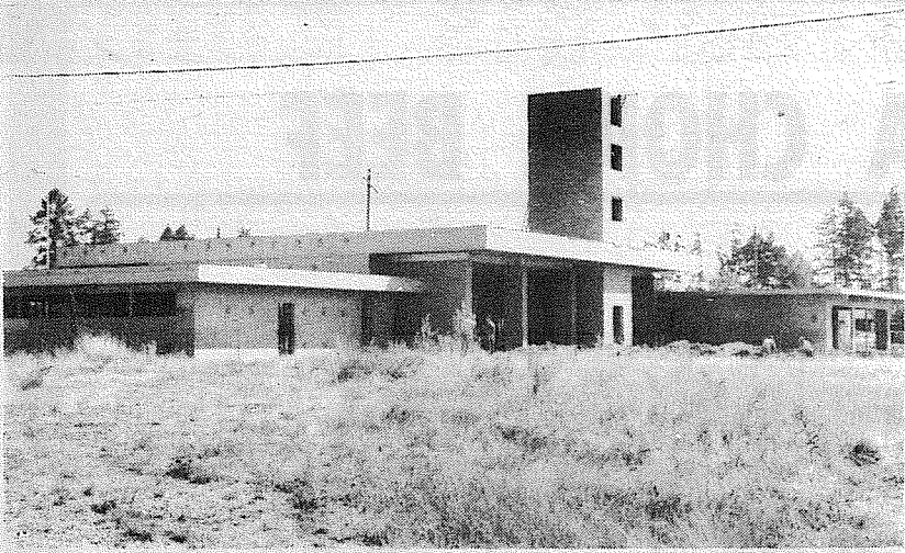
OCTOBER OCCUPANCY — The Parkland Fire Department is approximately seven weeks from completion released Ray Hixon, Chief of the department. The building has been running a little behind schedule because of technicalities, he said, but it is expected that the lost time will be caught up.
