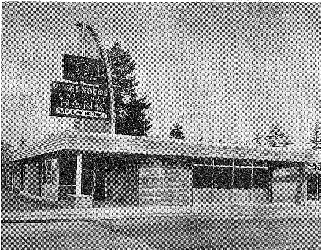
BIG STEP FORWARD —The handsome new bank building of the 84th and Pacific Branch of the Puget Sound National Bank is holding Open House Saturday, April 27. Manager Ralph Hubbard and staff moved to the new building over last weekend and were open for business Monday. An Open House is being held from 10 a. m. to six in the evening this coming Saturday. The public is cordially invited to attend.
