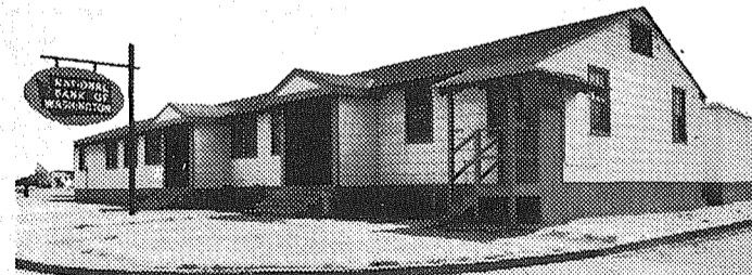
McChord A. F. Base Facility Building No. 609
