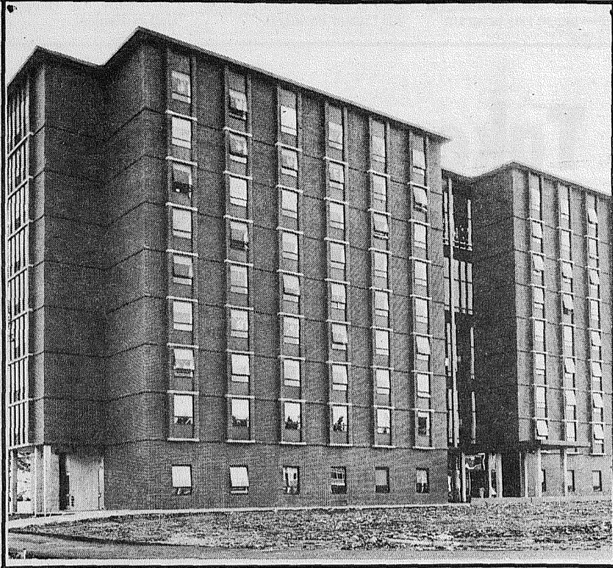
Tingelstad Hall, $2 million resident unit for 396 men.
