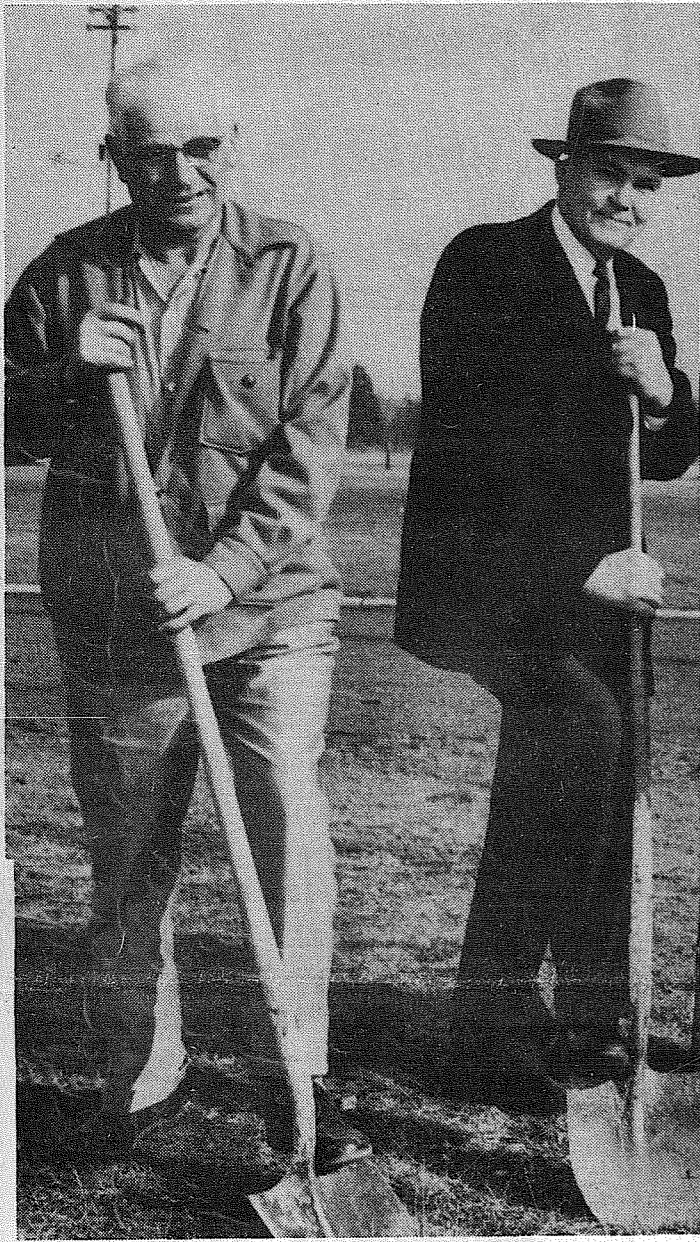
ART CRATE AND BOB MARTIN show what it takes to get a community moving on a worthwhile project—you just dig in! This is the start of the ground-breaking for the now completed Bethel Stadium which will get its first try-out at the Friday night game between Bethel and North Thurston. The Stadium will seat approximately 1500 and has a snack bar annex which will be operated by student organizations for fund raising projects.
