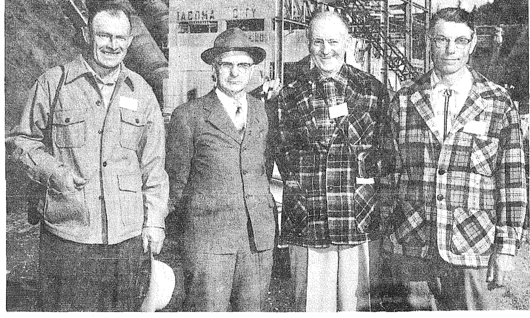
OFFICIALS of Parkland's Light and Water Co. and the Elmhurst Mutual Co. joined members of Tacoma's Public Utility Board and other leaders on a tour of the Cowlitz river development. Pictured at the construction area of Mayfield dam are, left to right: Alvin Raper, T. A. Lindgren and John Curtis, all of Parkland, and Harold LeMay of Elmhurst. The group is standing near the site of the powerhouse and in the far right
