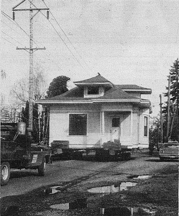
House movers have their problems as they struggle to move a house down C Street in Parkland. Overhead power lines would not move an inch from where they were, they just kept hanging there. Just mad with power we guess?
