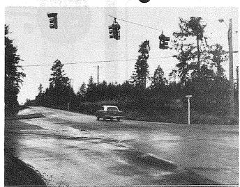
INTERSECTION SAFER-Looking north on Spanaway Loop Road at the intersection with Military Road, this is the look of the new traffic signals installed recently by the County. With timed signals, drive-over controls and free right turns, the intersection will be safer and easier to pass through for drivers using either road. -Times Journal Photo
