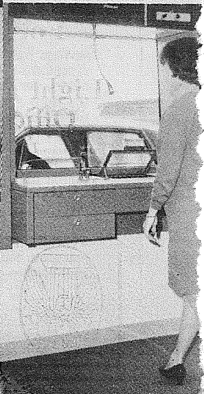
Interior view of the Drive-Up pay window.
