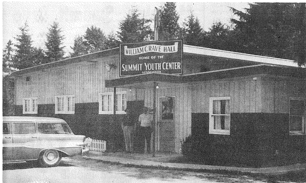
FUTURE IN DOUBT —William Rave and Sam Harris, two members of the Summit Youth Center Association, Inc., stands on the porch of the Youth Center Building on the grounds
