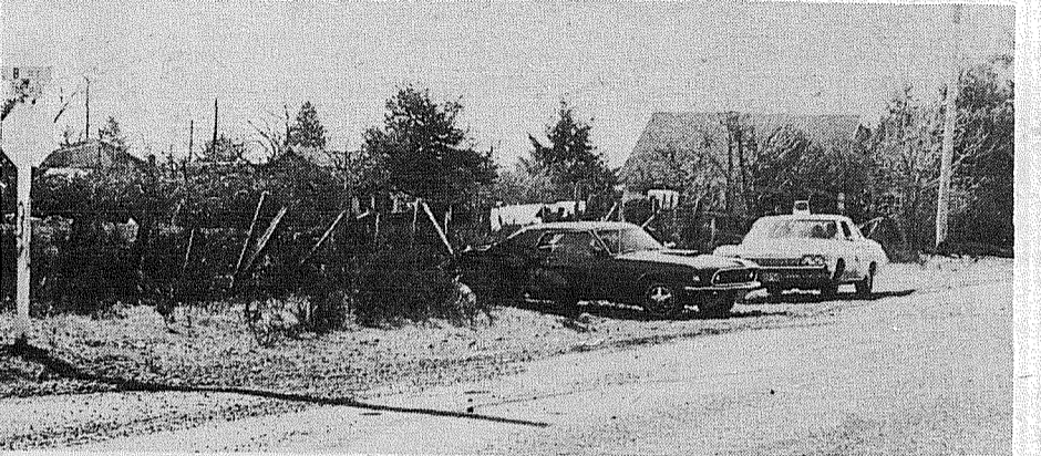
PASSENGERS IN THIS 1969 Mustang narrowly escaped serious injury when the vehicle ran into the path of a fully loaded dump truck at 168th and East "B" Sunday afternoon. The skids in the foreground were left as the driver of the truck, Robert Sulkosky of Puyallup, locked his brakes in an effort to avoid the Mustang driven by William Felter Jr., 22, of Tacoma. Evidence at the scene indicated that the difference between a severe accident and this minor traffic incident was measured in split seconds. If the impact had occurred a fraction of a second sooner the huge truck would have driven over the passenger vehicle.
