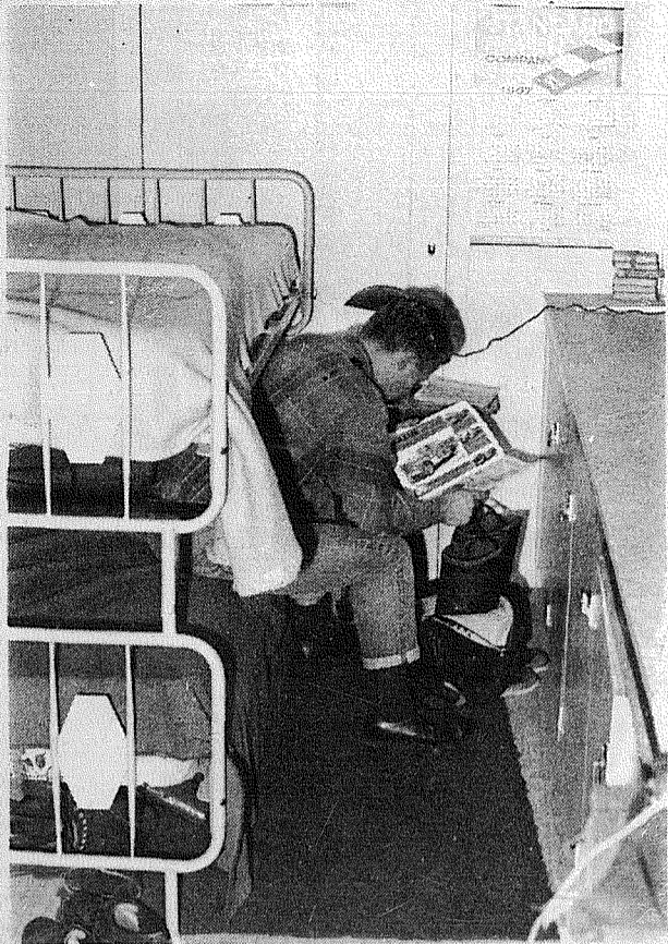
BROOM CLOSET DORM - Firefighter Gary Hauenstein, a live-in member of the Parkland Dept., shares his janitorial supply closet living quarters with work bench, tools, mop buckets, light bulb supply, and extra oxygen tanks. Holes drilled in door supply ventilation.
