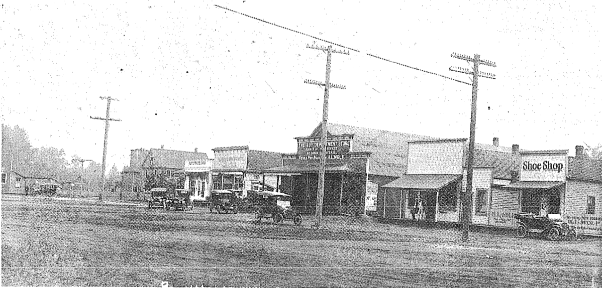
ENTIRE BLOCK pictured in this 1929 photograph of Roy Department Store. Business houses were wiped out by a fire that broke out in the attic of block one of McNaught's first addition to Roy.
