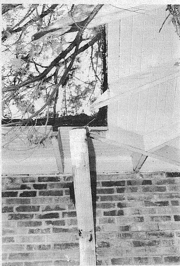
DRY ROT has completely destroyed exposed rafters causing gutters and drain pipe to drop to the ground. (Lower) Rusted drain pipe stands unattached to gutters, long since the victim of dry rot.
