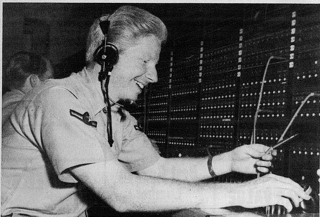
JIMMY BOYD, recording TV and motion picture star, operates the Base Communications' telephone switchboard as part of his two weeks training with that office. —Official USAF Photo
