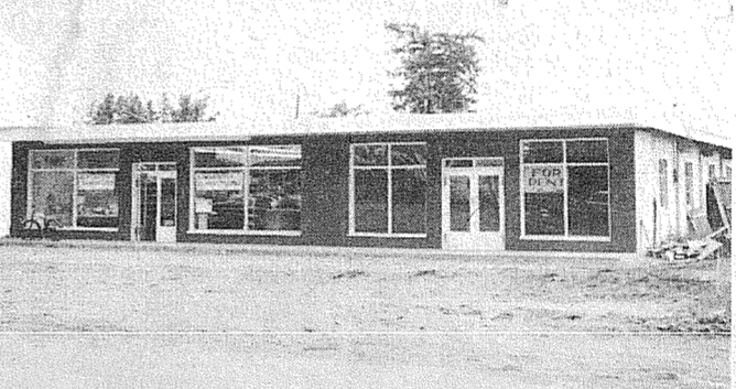
THIS IS THE NEW HOME of Ashmore Pharmacy on 166th and Pacific. The brick front building was built by Locke Construction, General Contractors. They have about twice the space that they had in their old building. Business is going on as usual while the final moving-in process is taking place.
