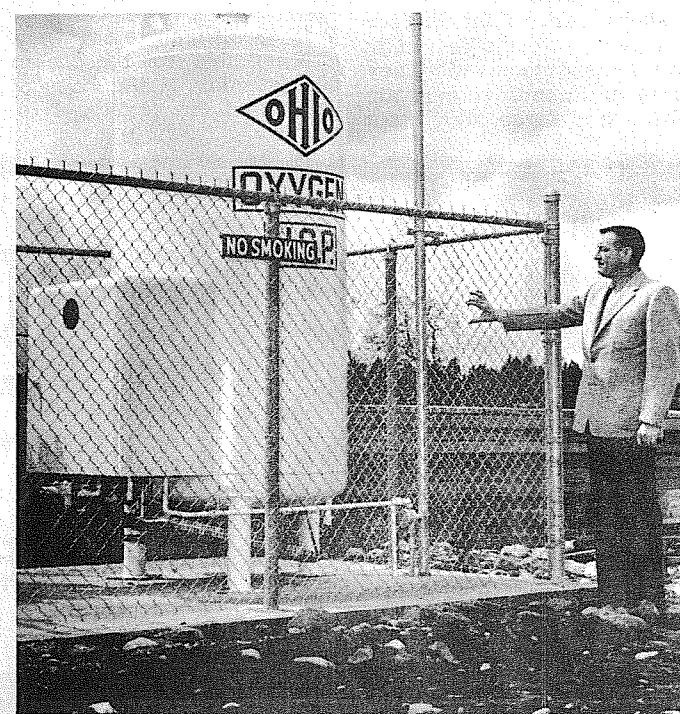
NEW SERVICE — Howard Hanlon, chief of plant operations, inspects the newly-painted 34,000 cubic foot capacity oxygen tank located behind the hospital. The tank will provide oxygen to every room in the hospital. TIMES Photo
