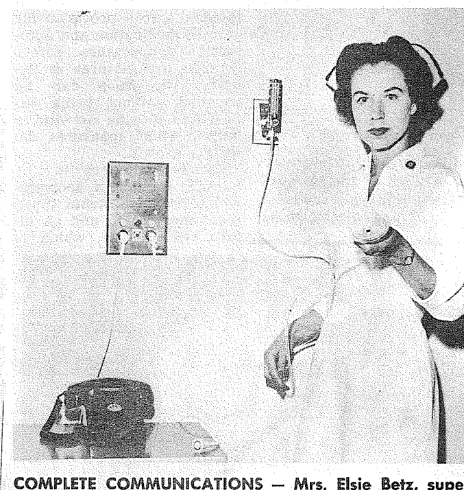
COMPLETE COMMUNICATIONS — Mrs. Elsie Betz, supervisor of medical service, demonstrates how oxygen would be provided from the wall outlet beside a patient's bed. The control panel to her left gives the patient instant communication with the nurse and has facilities for radio and television viewing. TIMES Photo
