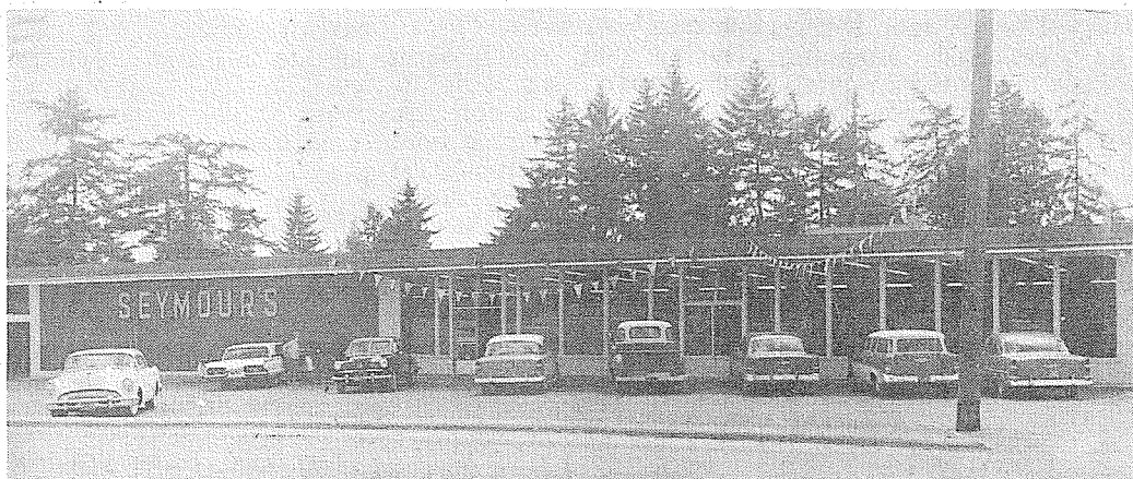
EXPANSION — This is the new look of Seymour's on Pacific Avenue since the addition to the building was completed recently. The added room gives the store almost double the previous
