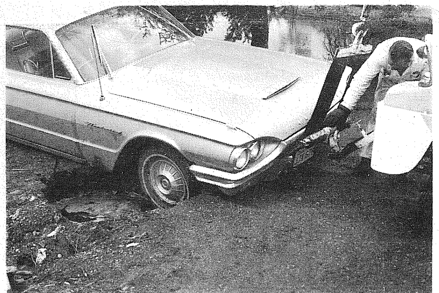
RAIN WASHOUT. Tow truck operators secure lines to the car belonging to Glenn Rogers, 610 East 112th, after it stalled in a hole about 2 feet in diameter and 5 feet deep that caved in as the vehicle was about to enter East 112th. Mrs. Rogers, who was driving, said the driveway culvert gave way as her car passed over it. Rogers blamed poor drainage of the area as the cause stating the roadside ditches frequently overflow flooding both his and his neighbors front and back yard after a heavy rain. The incident happened Monday morning. Numerous complaints to both the State Highway Department and County have resulted in little action, he said.
