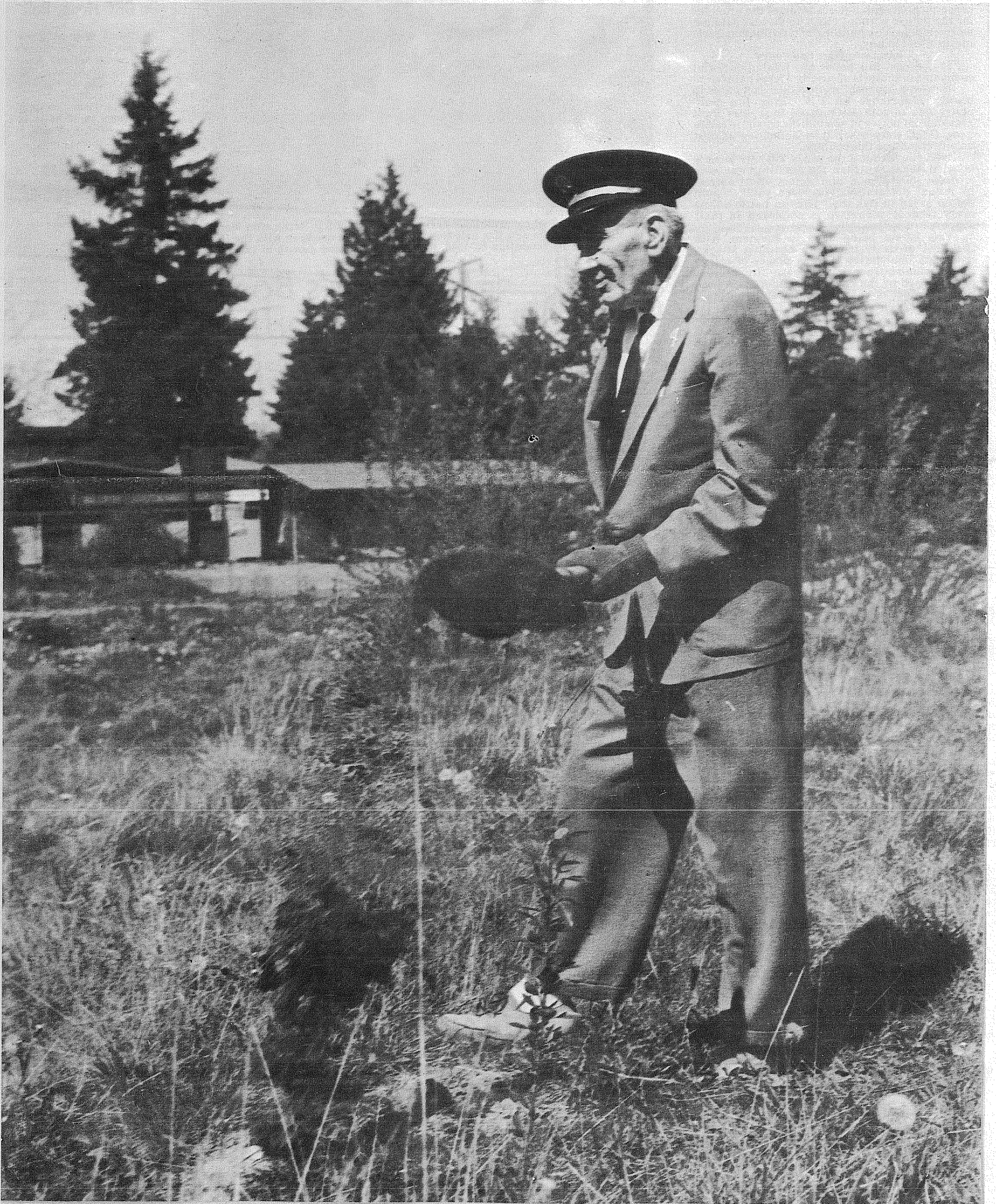
FIRE HALL GROUND-BREAKING. Clarence Marsh, charter member and one of first commissioners elected in Parkland Fire District, manned a shovel to break ground for the new $185,250 fire hall Monday. Contractor is George Yulleberg, Inc. See page two.
