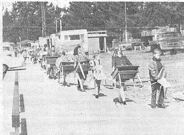
And the move goes on midst the hustle and bustle of construction crews.
