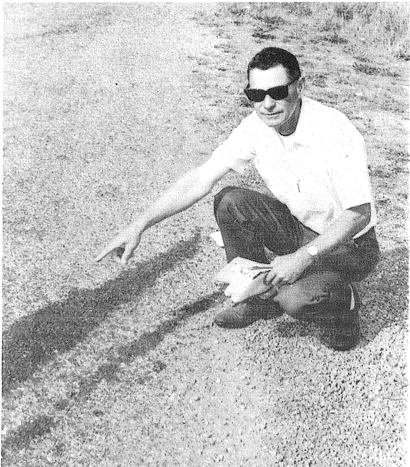
ELMHURST POWER and Light employee C.M. Jolly points out a trail of oil left by thieves who removed 3 transformers from the company premises earlier this week. Oil dripping from the get-a-way vehicle led employees and Sheriff's Deputies to recovery of the property at an isolated area near 72nd and Waller Road.
