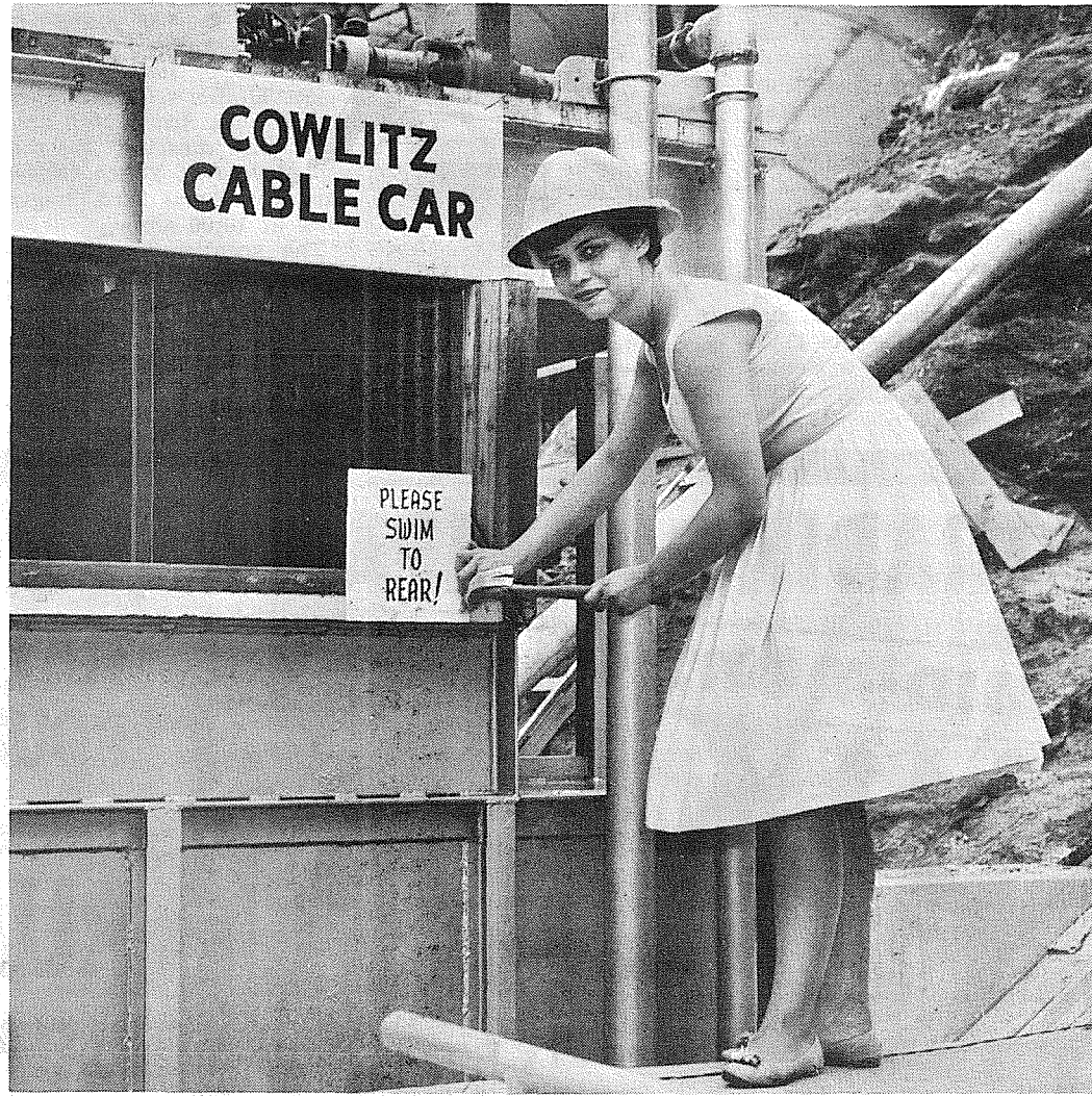
GOING UP? COWLITZ CABLE CAR. This cable car device gives fish a free ride from the end of the fish ladder at Mayfield Dam to top of
