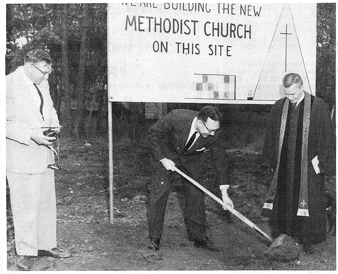
GROUND-BREAKING —Lloyd Carey, left, building committee chairman, looks on as Rev. Wischmeier, Methodist District Superintendent, turns a spadefull of ground at the ceremony for the new Spanaway Methodist Church. Rev. Qualley, pastor of the church, conducted the special service on Sunday. —Photo by Dugan
