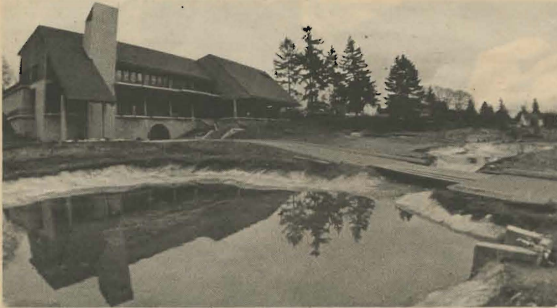
Lake Wiegman is a thinking man's pond, for one must ponder the faults of waltzing asphalt which looms like a marooned oil spill in man's attempt at naturalness.
