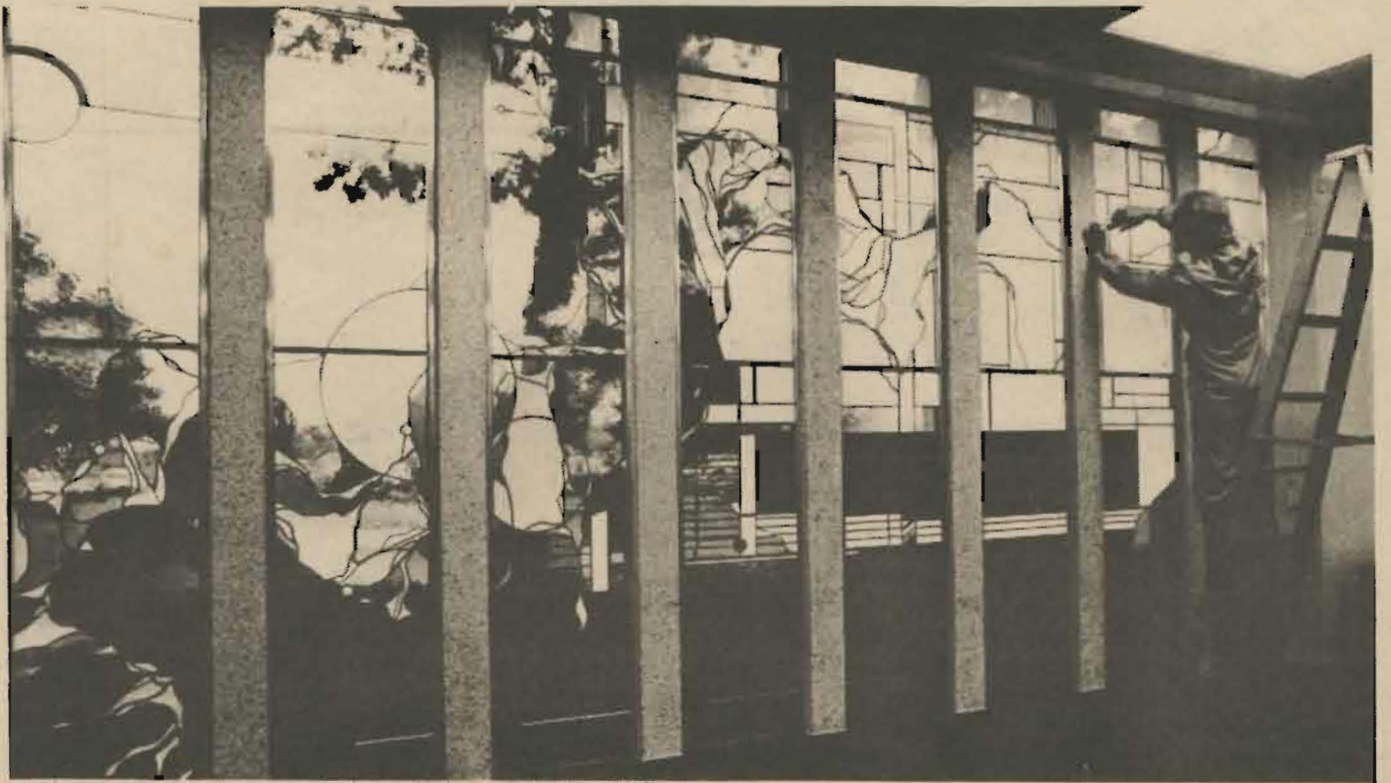
Mark Gulsrud installs new art glass window at Mortvedt Library.
