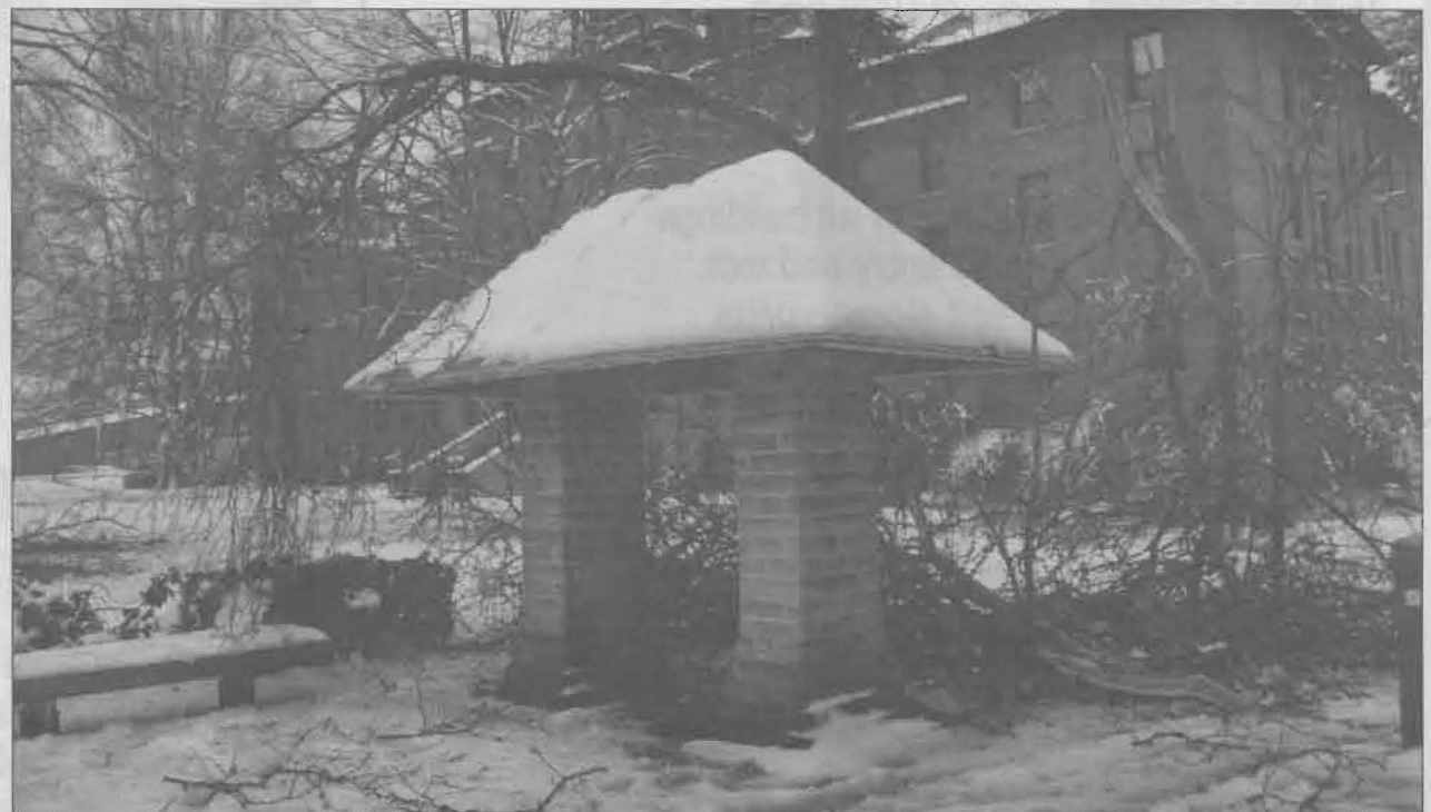
Damage due to the ice storm extended from the pool on lower campus to the Women's Center on upper campus, scattering debris across the grounds. Trees and fallen branches from the storm will be used in various projects, but the trees will not be removed from campus until their replacements are planted.
