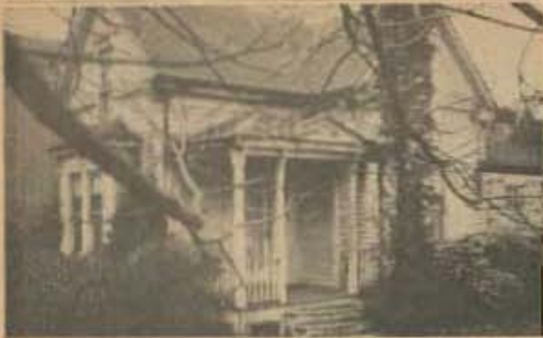
COMING DOWN—Another part of the PLU "phase it out" program will get underway June 1st. The largely old frame located 30 feet east of the Administration Building was recently purchased by the University for what university officials term "a fair market price."
