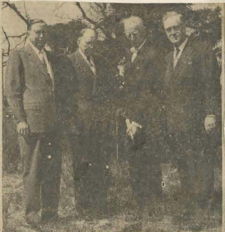
PLC Groundbreaking —Ground was broken Friday for the college union building on the Pacific Lutheran College campus. Dr. J. C. K. Preus of Minneapolis, with shovel, is shown as he turned the first spadeful of earth. Others pictured are, left to right, Dr. Philip E. Hauge, dean of the college; the Rev. O. K. Davidson, Tacoma, secretary of the college board; Dr. S. C. Eastvold, president of PLC.
