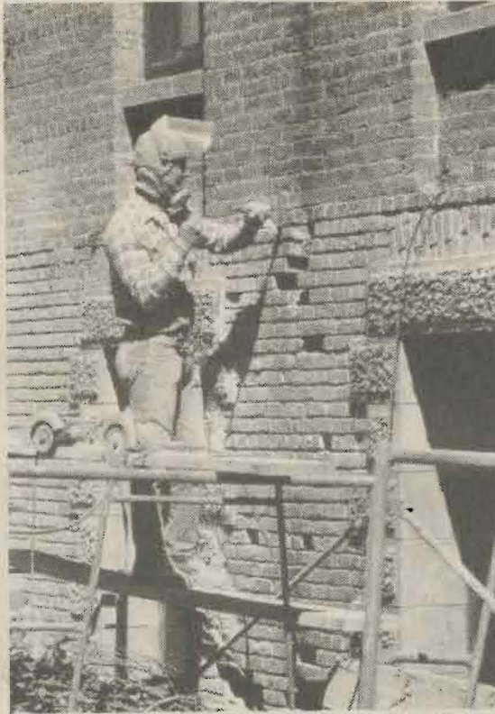
Each brick in Harstad Hall was "repointed" and defective mortar replaced.
