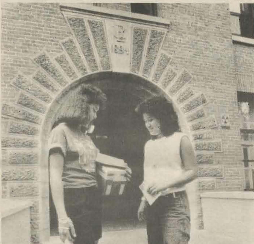
Removal of Harstad Hall ivy revealed a 91-year-old PLU logo above the building entrance.
