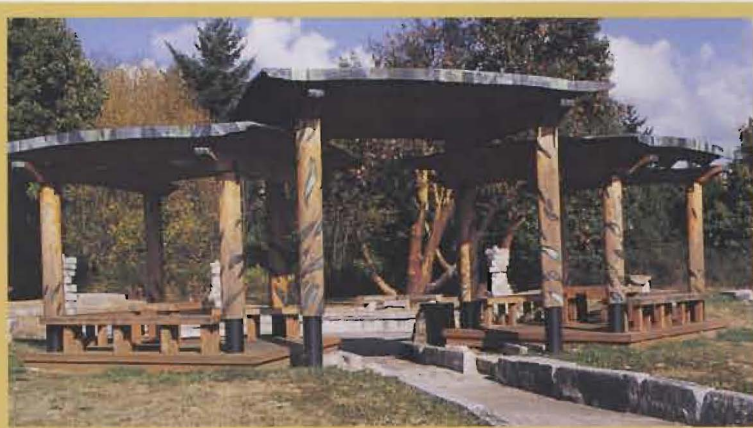
Weddings, prayer services and community events are held at this gathering place at Salishan. It was built with salvaged materials from the city of Tacoma, including copper from the original dome of Union Station.
