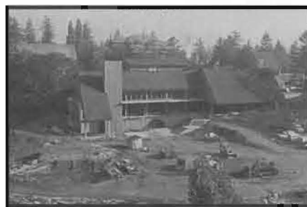
The University Center under construction in 1970.
