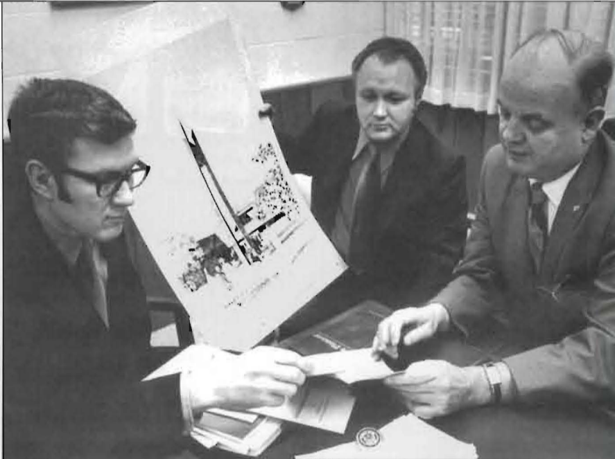
EARLY DEVELOPMENT: In 1971 (l to r) David Berntsen, Edgar Larson, and Clayton Peterson review drawings of the proposed 60-foot Anderson Clock Tower outside the University Center that was erected later that year. The tower was the gift of Herman '31 and Vivian Anderson. Today Berntsen and Larson continue to serve as development officers for the university.
