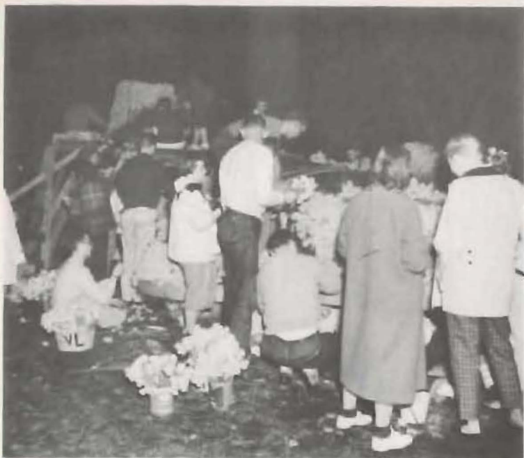
Construction continues late into the night.
