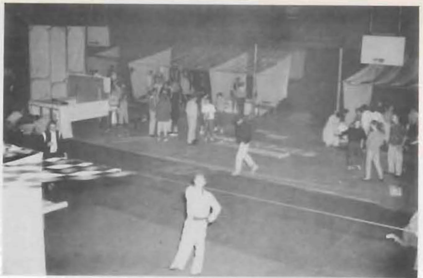
Construction activity gets into full swing.
