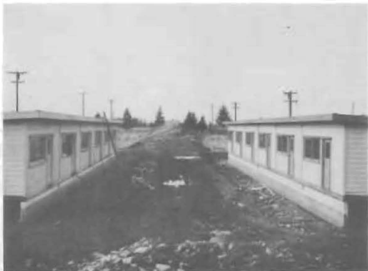
Construction begins on new men's housing unit, Evergreen Court.
