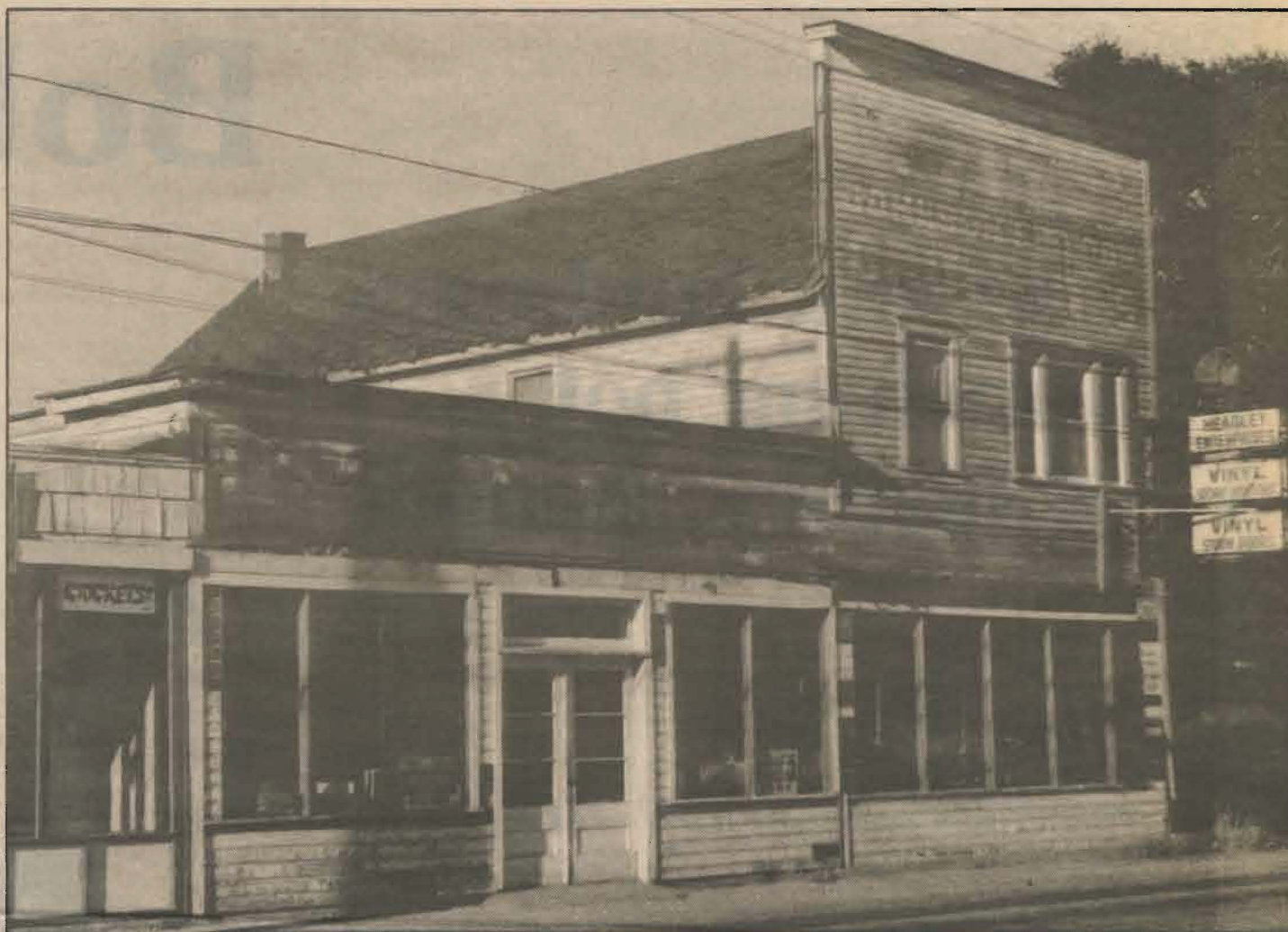
This Garfield Street building is one of the targets of the Parkland revitalization program. Saturday's festival was an effort to call attention to the Parkland community.
