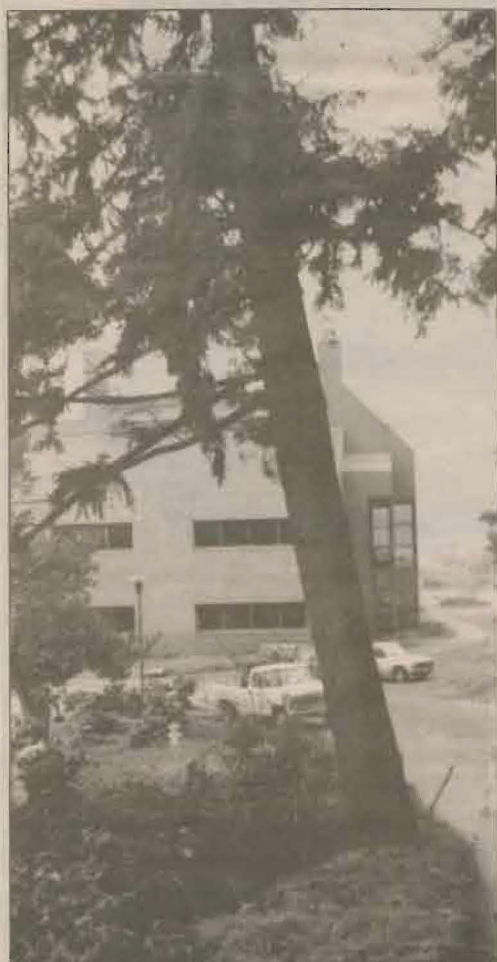
Rainy weather and winds last week caused this tree behind Hinderlie Hall to start leaning toward Foss Field.
