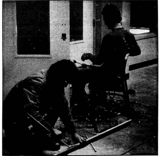
Workers are finishing PLU's remodeling project in Ingram Hall.
