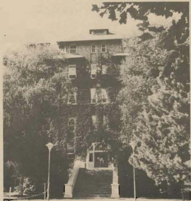
Harstad Hall (original Old Main)
