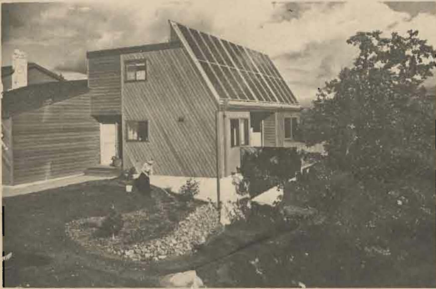
Boleyn's new solar house
