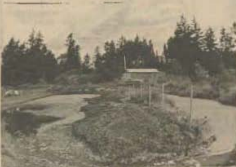
An encompassing view of the entire PLU sewer system leaves something to be desired.
