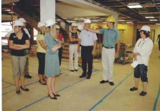
Tom Huelsbeck, director of residential life, highlights changes to the University Center during a tour of the remodeled building.
