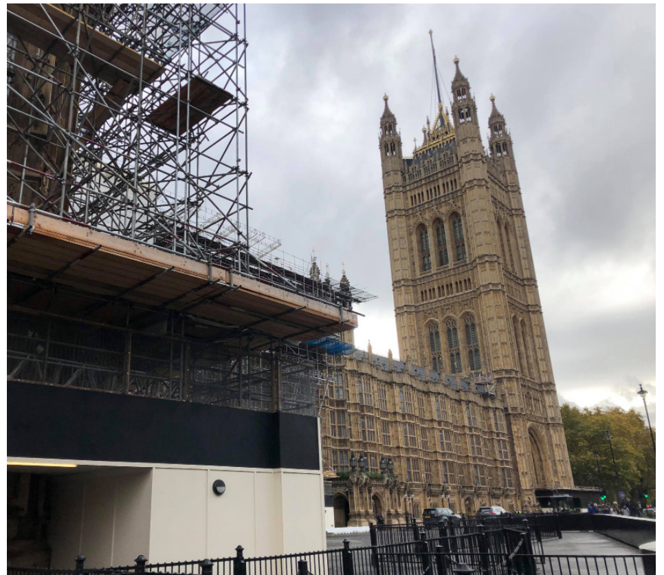
Image of Westminster Palace under scaffolding. Photo by Gurjot Kang.
